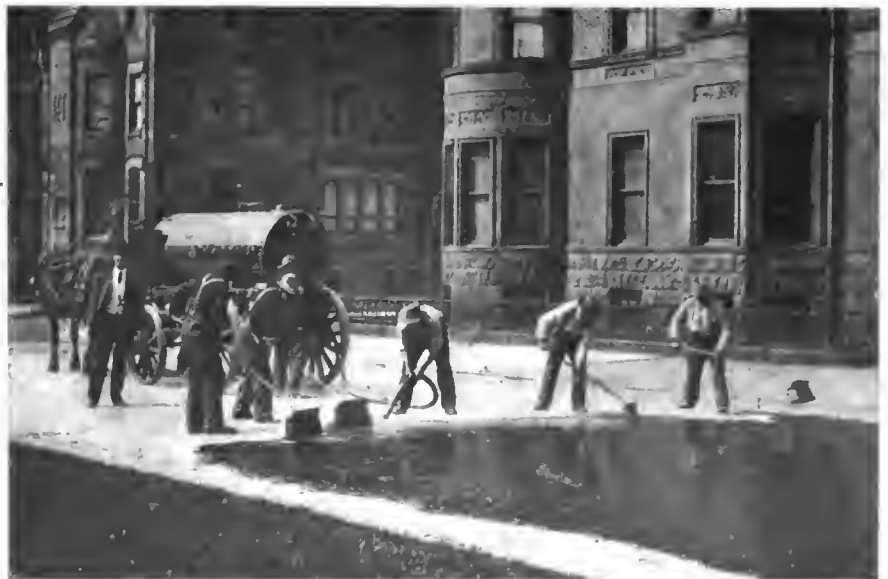
SPREADING TARVIA ON COMMONWEALTH AVENUE, BOSTON.
